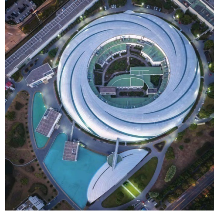
Fig. 1 A view of Shanghai Synchrotron Radiation Facility [7].
