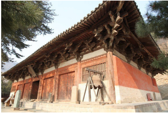
Fig. 11 The Main Hall of Foguang Monastery [7]
